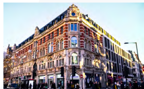
工商大廈 Industrial and Commercial Buildings
