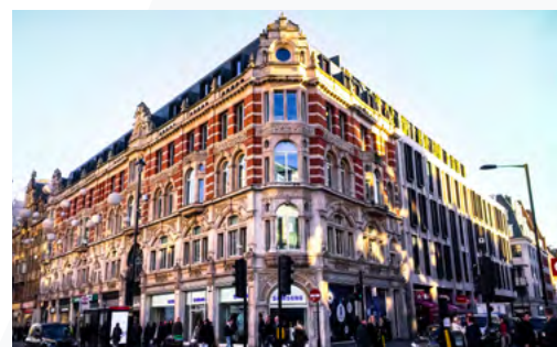
工商大廈 Industrial and Commercial Buildings
