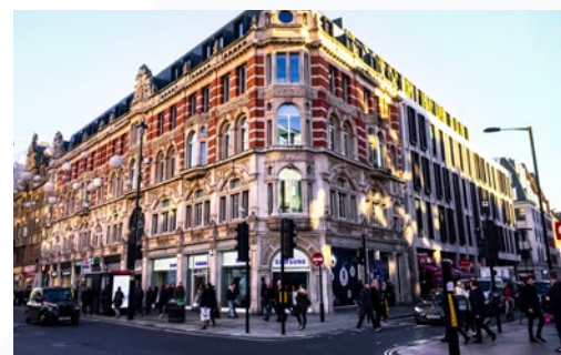
工商大厦 Industrial and Commercial Buildings
